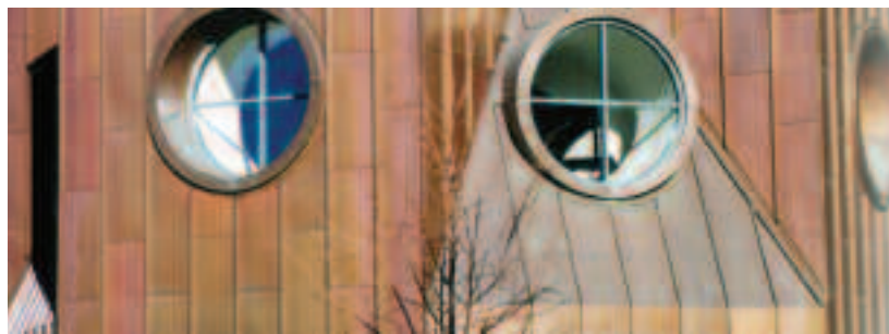
Figure 7 — Batten seam panels on the Denver Library Children's Pavilion illustrate one new use for architectural copper other than roofing.
