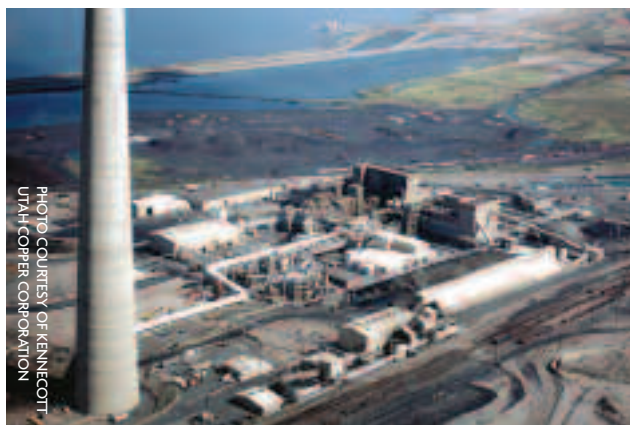
PHOTO COURTESY OF KENNECOTT UTAH COPPER CORPORATION Figure 1 — Modern copper smelters such as Kennecott Utah Copper's plant shown here remove more than 99 percent of sulfur released during smelting, converting it to sulfuric acid for use in leach/solvent extraction/electrowon operations.
