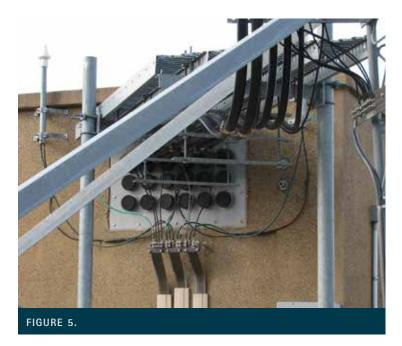
When lightning strikes one of the nine auxiliary sites that the county operates, energy is bled off the coax on the vertical run (Fig. 7), the coax where it penetrates the firewall (see above), and the interior side of the firewall (Fig 9).
