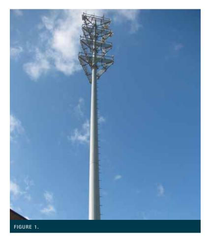
The COMTEC center's transmission tower was grounded when built, but age and corrosion had deteriorated the connections. Upgrades during restoration of the center included exothermically welded connections, new grounding electrodes and a buried copper ring ground.
