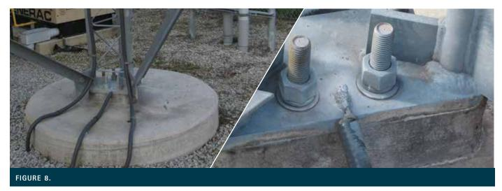
The photo on the right shows the reliable, exothermically welded grounding connection to the center cable, which connects the tower's steel structure to a buried bare-copper ring ground surrounding the tower and to the interior grounding bar shown in Figure 9.
