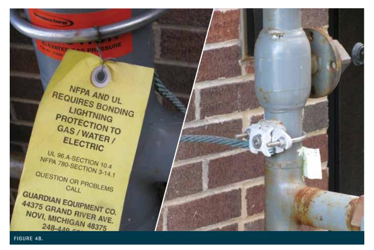
Grounding of the center's water and gas service entrances is provided by the heavy-gage copper cable, right. The tag shown on the left alerts technicians that grounding to gas and other services is code-mandated.
