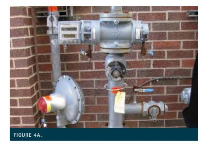
A proper grounding cable connection to a gas service line. The silvery, copper-alloy, UL-approved cable clamp is cadmium plated to prolong corrosion resistance.
