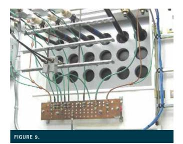
The facility's interior grounding bar is located on the inside of an exterior wall, immediately below penetrations for cables from the tower. Various green wires connect to those cables and to other grounding bars at the facility.
