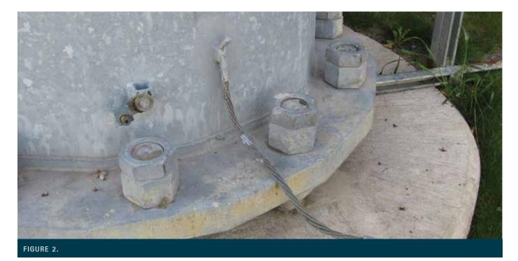
Tower-grounding cables were originally bonded with mechanical clamps such as the one shown at the far left foreground, but age and corrosion had loosened the connections, raising ground resistance. The facility upgrade included replacing those connections with exothermically welded bonds and 28R Class II lightning conductor cable, center.
