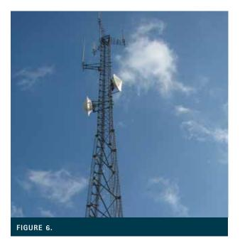
One of several auxiliary transmission towers operated by Macomb County. The towers extend emergency communications well beyond the range of the COMTEC headquarters tower. All towers are equipped with the same high-quality, all-copper grounding systems as those installed at COMTEC.
