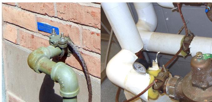
Figure 3. Braided lightning conductor (29 strands of bare 17-gage copper) is shown bonded to the fire station's water supply line, left. Note the use of UL96-approved copper alloy mechanical clamps. The clamps resist loosening and corrosion. Similar connections were applied inside the building.
