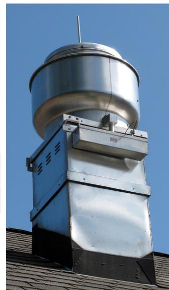
Figure 2. Rooftop ventilator with air-terminal. The otherwise ungrounded ventilator is within a six-foot strike distance of the lightning protection system's cabling (not shown) and is therefore connected to it.
