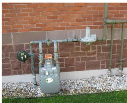
Figure 4. Ground Connection to Gas Service Entrance. The gas service and all exterior metal pipes are connected via the ring ground.
