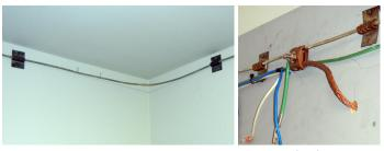
Figure 6. Halo ground installed around interior walls (left) to facilitate connections to electrical, telephone and electronic equipment, cabinet racks and wall penetrations, (right). Note the generous size of the braided lightning cable entering from lower left.
