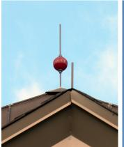
Figure 1. Air terminals (strike termination devices) are mounted at a code-mandated maximum 20-ft interval on the roof of the Simsbury Main Station No. 1. The decorative terminal is one of several installed for architectural reasons. Note the braided copper lightning conductors mounted along gable edges.
