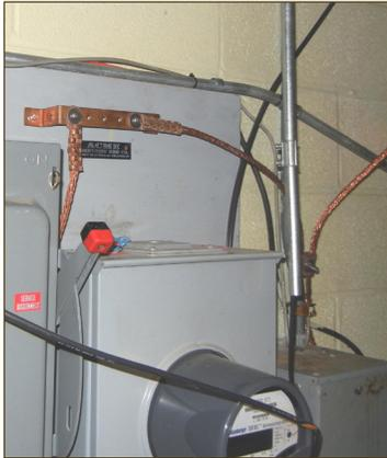
*Figure 10. Upper photo: grounding conductors run along walls and from room to room in the venerable fire station. Lower photo: a copper ground bar serves as the ground-to-lightning system bus at the station's service entrance. Note that braided copper lightning cable extends all the way to the service entrance.*
