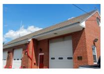
Figure 8. View of the Wethersfield, Connecticut Fire Station No. 2, one of the oldest in the state. The tower behind the station at far left serves the station's communication needs. Air terminals are spaced at 20-ft increments along the roof ridge line.
