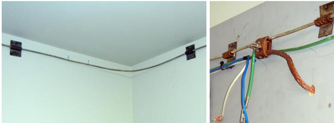
**Figure 6. Halo ground installed around interior walls (left) to facilitate connections to electrical, telephone and electronic equipment, cabinet racks and wall penetrations, (right). Note the generous size of the braided lightning cable entering from lower left.**
