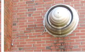
Figure 9. Left, the braided copper down-conductor is well-concealed, and extends from the rooftop to a driven 10-ft electrode later covered by concrete. The ventilator (Fig. 9, right), being connected to a metal system, is bonded to this down-conductor.
