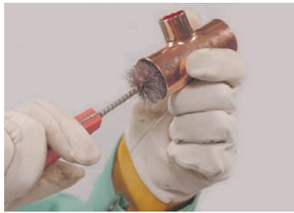
Fig. 5 — Fitting cups must also be cleaned.
