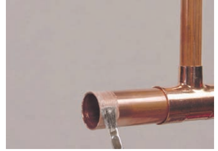
Fig. 6 — Flux is applied to the tube soon after cleaning.
