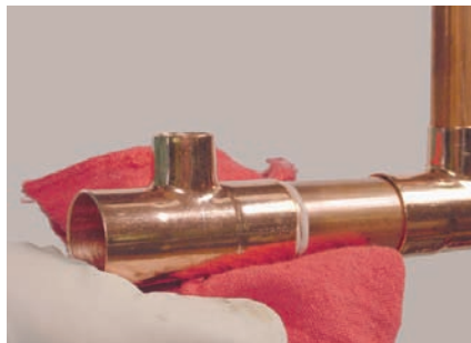
Fig. 8 — Excess flux must be removed.
