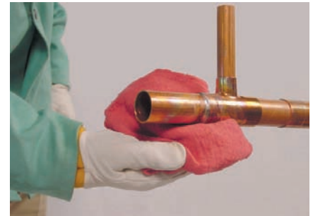
Fig. 12 — After cooling, clean off any flux residue.
