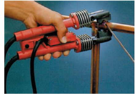
Fig. 11 — Heat can also be applied with an electric resistance soldering tool.
