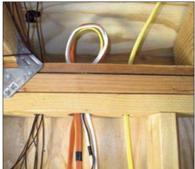
Figure 3. Bundle of 6 NM-B cables installed in top plate
