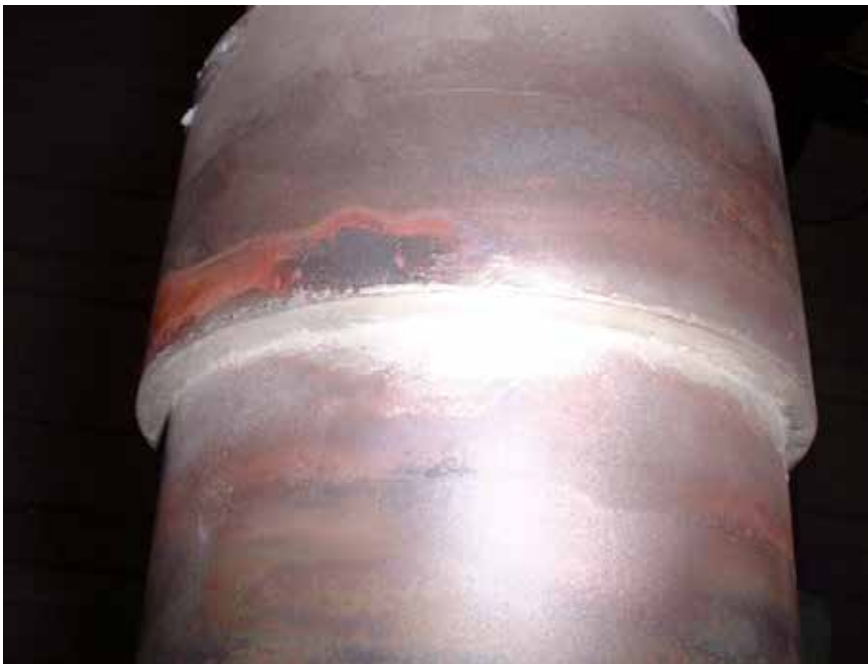
Capillary brazing of a sleeve to a pipe using a silver solder. (Courtesy Eucaro Buntmetall GmbH)
