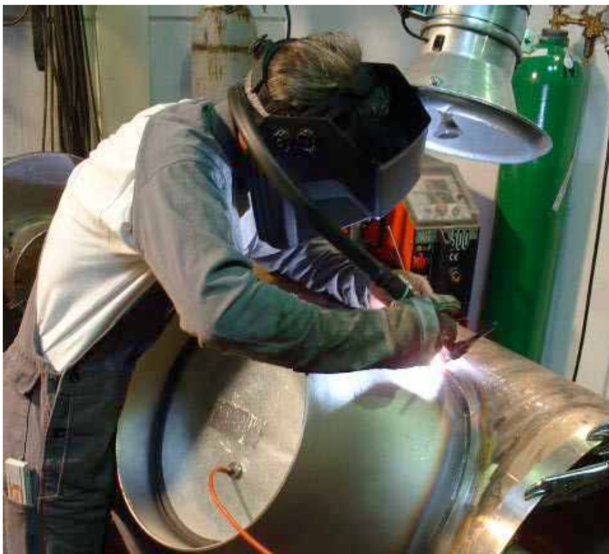
TIG (GTAW) welding 90-10 copper-nickel assembly. Note baffle for backing gas supply at root run stage (Courtesy Eucaro Buntmetall GmbH)
