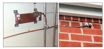
Figure 6. Indoor grounding bus with wall penetration (left); the right-hand photo shows one of several outdoor wall penetrations, from which the heavy-gage copper conductor to the left of the penetration lug leads downward to a driven earthing electrode.
