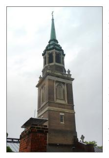
Figure 8. St. James's 160ft, copper-clad steeple stands at the front of the church. Although a 1994 lightning strike probably hit the steeple, destroying the church, the steeple itself remained relatively unharmed. The steeple was not grounded before the lightning strike. Now, the steeple, the periphery of the church's roof and all rooftop equipment are protected by strike termination devices (Franklin terminals), all bonded to a securely grounded, 100% copper lightning protection system.
