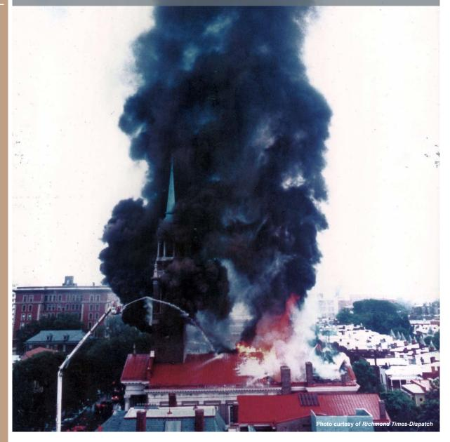
The near-total destruction of Richmond, Virginia's historic St. James Episcopal Church by a 1994 lightning strike is believed to have resulted when the strike hit the ungrounded, copper-clad steeple, from which energy traversed the wooden roof structure, setting it ablaze, rather than being directed safely to earth. An alternative explanation sees the strike initially contacting a distribution transformer behind the structure.
