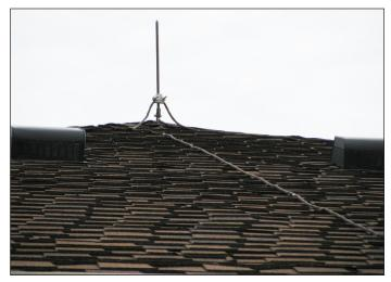
Figure 4. The weathered copper down-conductor leading from the Franklin terminal on one of the church's two towers blends well against the roof's reddish shingles. Attention to aesthetic details such as this helps make externally mounted lightning protection system components unobtrusive elements of the building's appearance.
