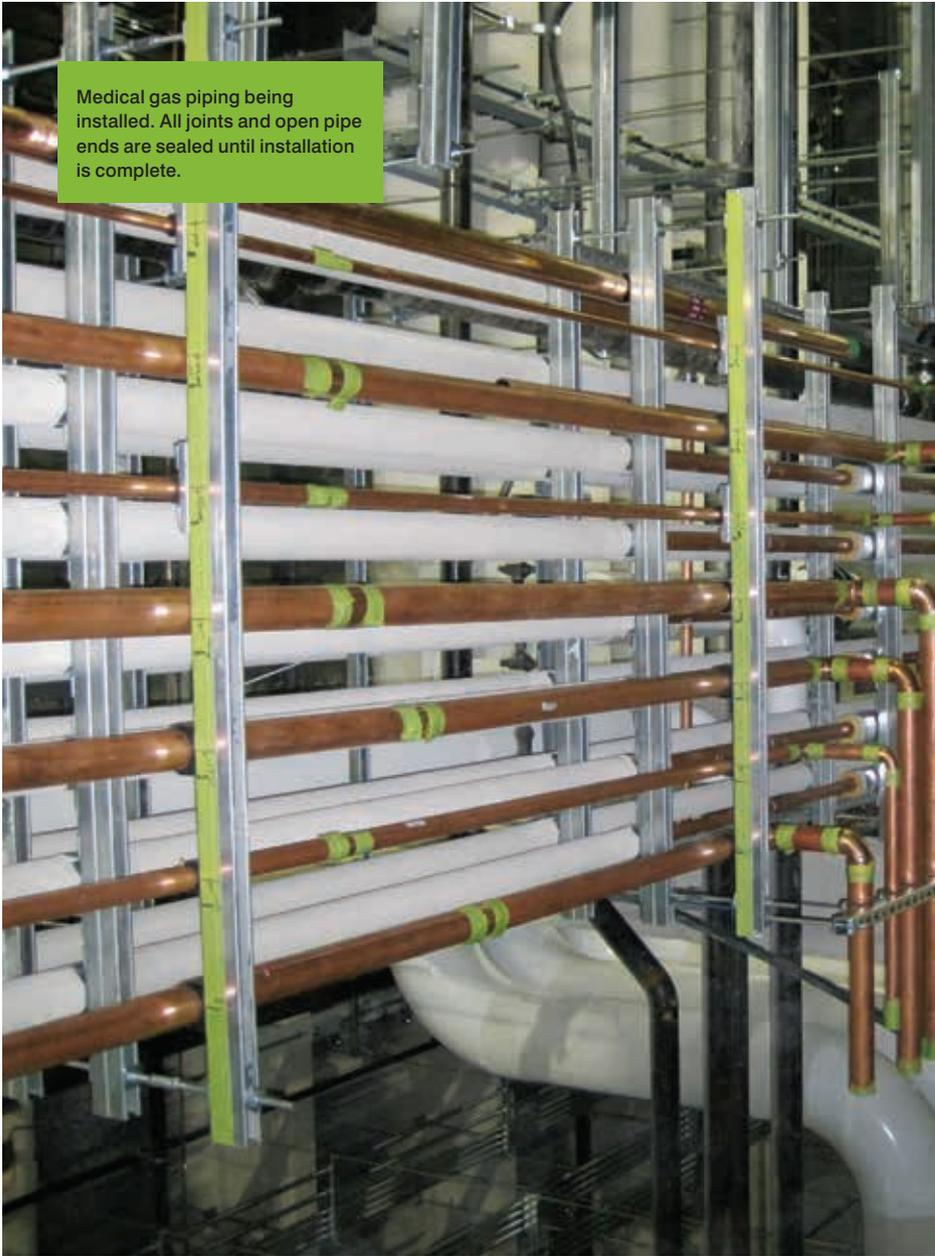
Medical gas piping being installed. All joints and open pipe ends are sealed until installation is complete.
