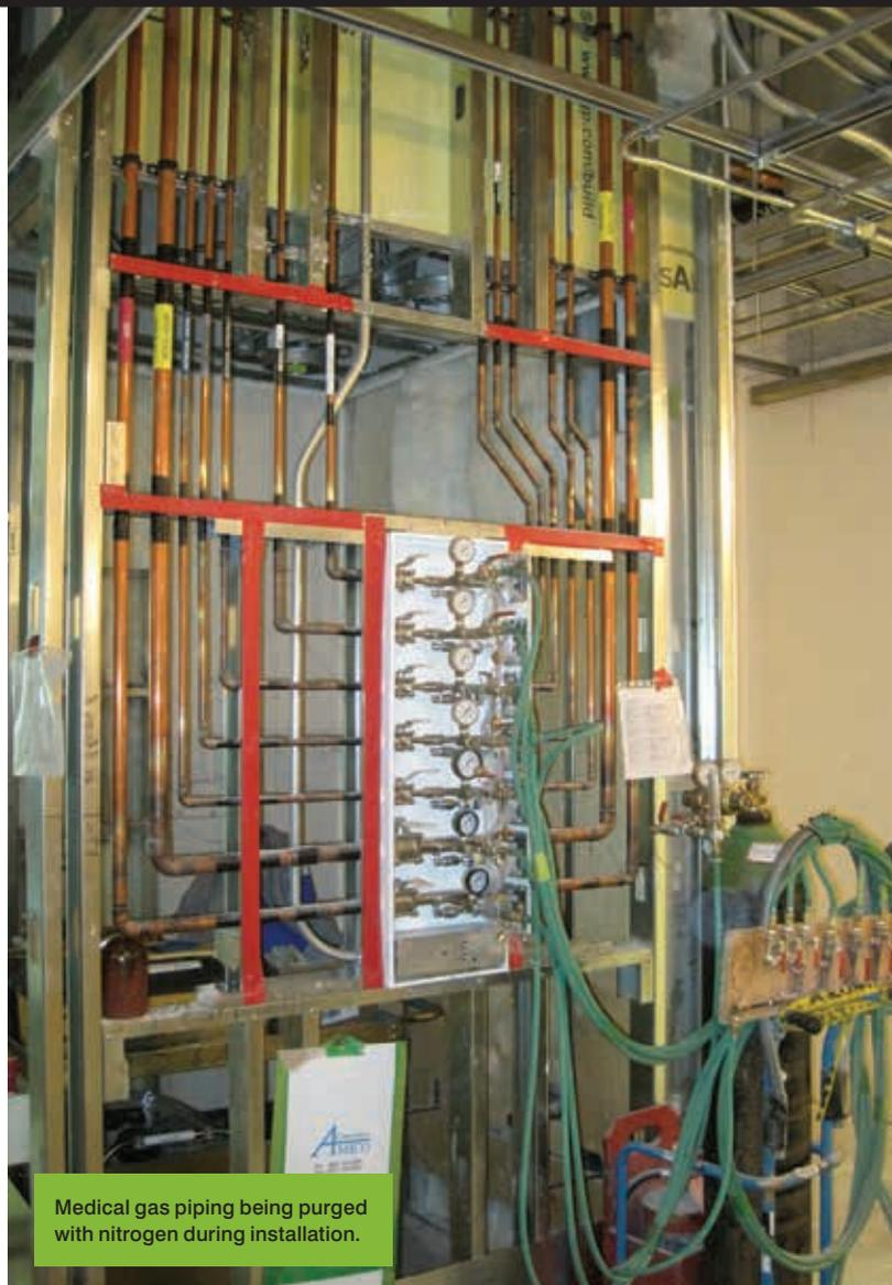
Medical gas piping being purged with nitrogen during installation.
