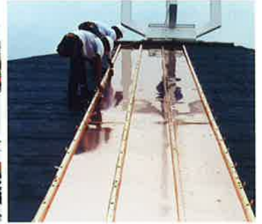
At left: Initial weathering can be swift and uneven, sometimes depending on undetectable factors such as mill lubricants. Fear not: it all evens out in about a year; studies show. Center, handling coils for site roll forming. At right, a traditional batten seam installation on a North Carolina church. PHOTOS: LEFT, SHANE JOHNSON; CENTER AND RIGHT, PICKARD ROOFING
