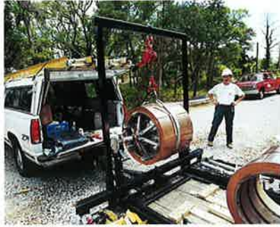
At left: Initial weathering can be swift and uneven, sometimes depending on undetectable factors such as mill lubricants. Fear not: it all evens out in about a year; studies show. Center, handling coils for site roll forming. At right, a traditional batten seam installation on a North Carolina church. PHOTOS: LEFT, SHANE JOHNSON; CENTER AND RIGHT, PICKARD ROOFING
