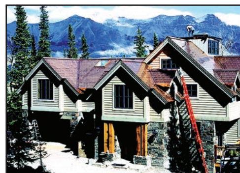
Known for its beauty, ease-of-installation, long lifespan and high performance in extreme weather conditions, copper shingles are becoming a popular roofing material, especially among high-end homeowners. Photo Courtesy of Revere Copper Products
