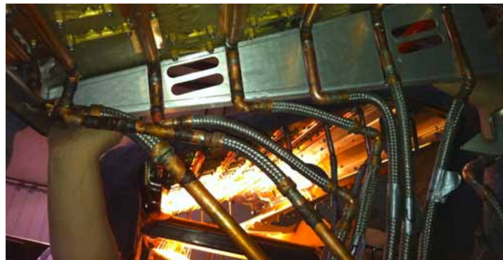
Copper tubing installation at the 9/11 Memorial – Credit Ronaldo Vega
