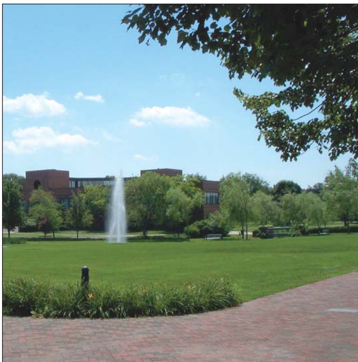
Figure 1. Energy savings are a top priority at Bryant University. Regional energy costs are higher than the national average, but high-efficiency NEMA Premium® motors help keep costs down, while a 100% copper electrical system provides high power quality for the school's extensive computer and communications facilities.
