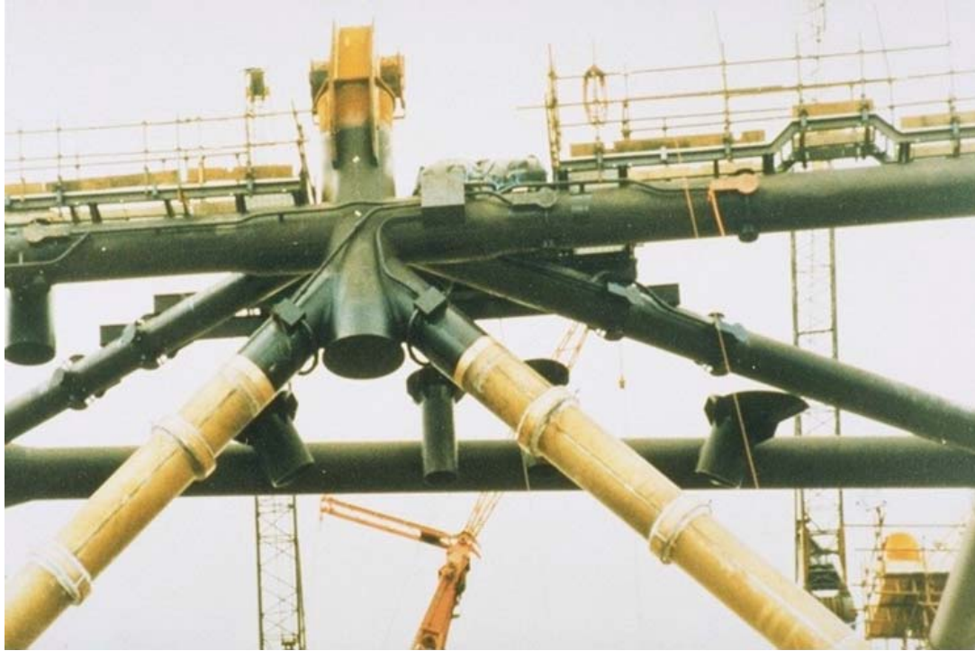
Figure 4. Cu-Ni sheathing applied to a Morecambe Field Structure
