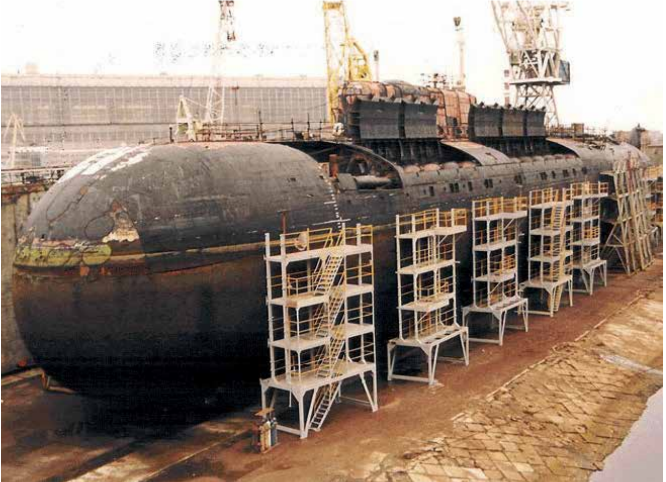
Figure 17 - Dismantling Oscar 1 Class Submarine (Courtesy Keel Marine Ltd)
