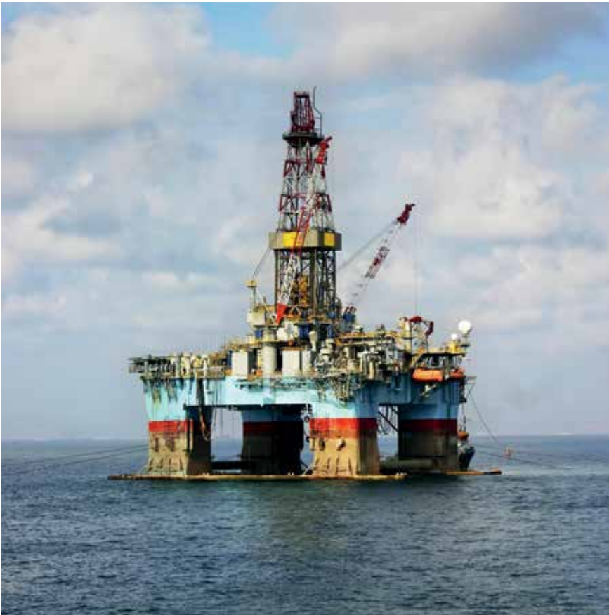
Figure 12 - Between 150-200 tons of 90-10 copper-nickel have been installed on individual drill ships for the fire fighting system (Courtesy KME Germany AG & Co KG)
