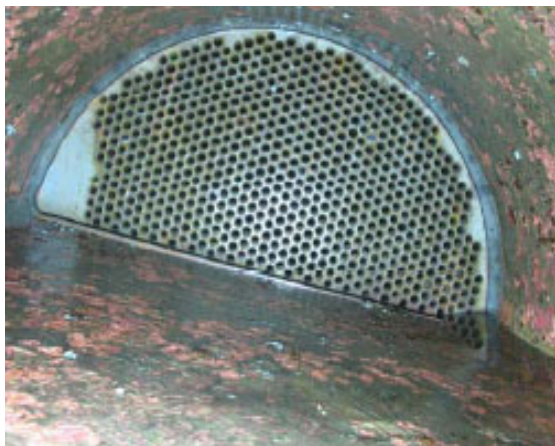
Fig 4 View as Fig 2 following chemical clean and debris removal (tubeplate diameter 850mm)
