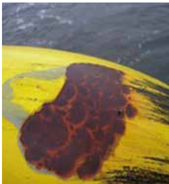
The 3rd coating layer of the transition piece, boatlanding and j-tube damaged due to tie-up of the service ships.
