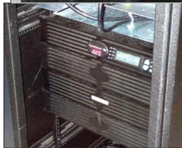
Figure 3. Server racks located in the Bello Center. The entire campus is networked from this location, for which power quality is maintained at the highest possible level by adherence to IEEE Recommended Practices. An uninterruptible power supply (lower photo) protects the network in the event of unscheduled outages.
