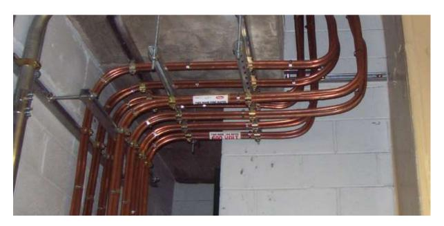
Pyrotenax MI Cable System 1850 from Pentair Thermal Management for use in System No. FHIT.1850 when installed in accordance with manufacturer's installation instructions dated December 2012. Applications include fire alarm wiring as well as wiring for other for critical lifesafety circuits in high-rise buildings, subways, tunnels, airports and health care facilities.
