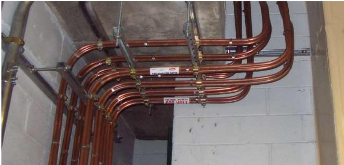
Pyrotenax MI Cable System 1850 from Pentair Thermal Management for use in System No. FHIT.1850 when installed in accordance with manufacturer's installation instructions dated December 2012. Applications include fire alarm wiring as well as wiring for other for critical life-safety circuits in high-rise buildings, subways, tunnels, airports and health care facilities.
