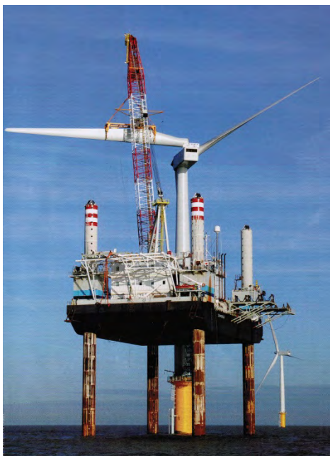
Figure 7. A large mast-mounted turbine being installed in the Irish Sea.
