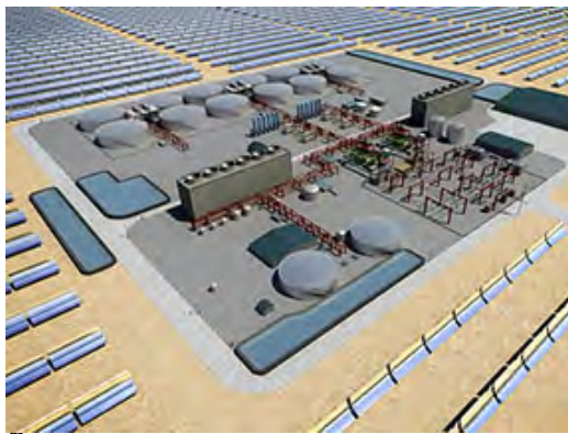
Figure 10. The 200+ MW Solana Solar Farm in central Arizona. It incorporates conventional trough-type collectors for steam generation along with molten salt storage for operation on cloudy days and at night.
