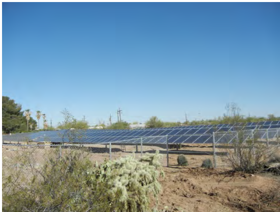
Figure 9. A 140-kW commercial-scale PV farm under construction. It will supply power to a water-utility office and garage. Installations of this type are one example of distributed generation.
