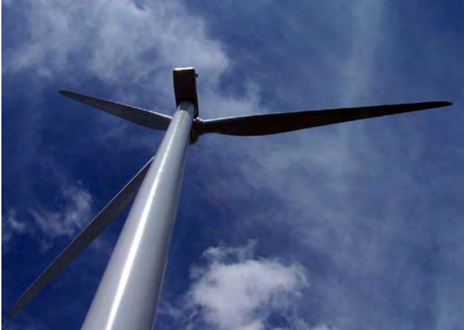
Figure 1. A contemporary three-bladed wind turbine showing its nacelle containing the gearbox and generator.
