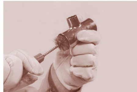
Figure 5. Cleaning: Fitting Brush
