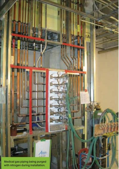
oxygen analyzer per section 5.1.10.4.5.5 of NFPA 99-15.
