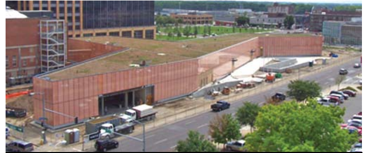
The copper sandwiched in the exterior glass walls of the new library in Des Moines will retain the appeal of its original color and sheen because it is protected from the atmosphere preventing patination.
