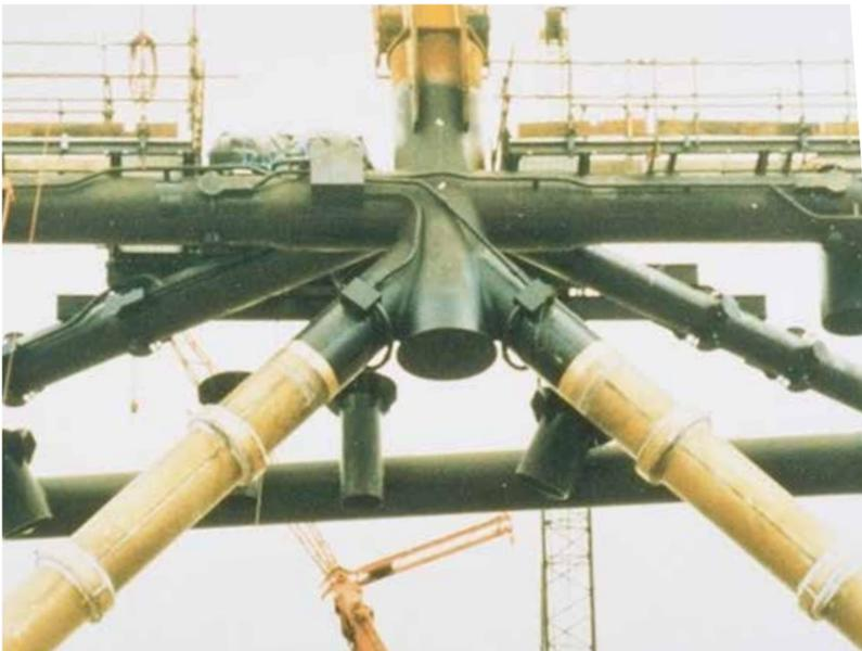
Structural members sheathed in 90-10 copper-nickel during construction of the Phase 1 Morecambe gas field platforms
