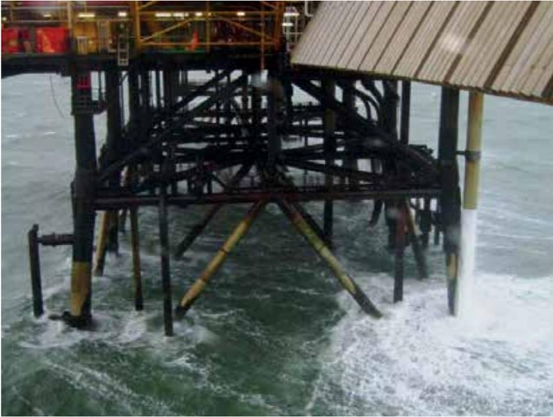
90-10 copper-nickel splash zone protection on a platform in the Morecambe Field, UK. The sheathing has been in service over 25 years
