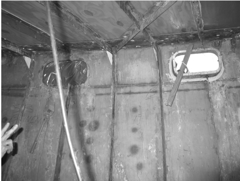
FIGURE 9: Inside of unpainted hull, showing hull plate, ribs and deck beams
