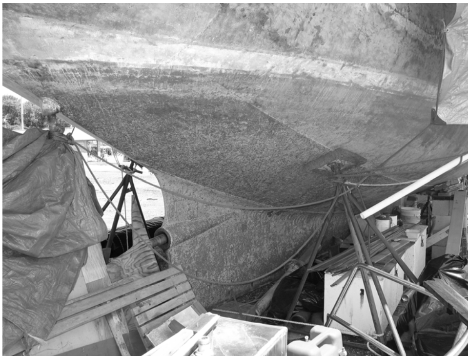
FIGURE 8: Stern, starboard side, showing trailing end of the keel and the web connecting hull to keel
