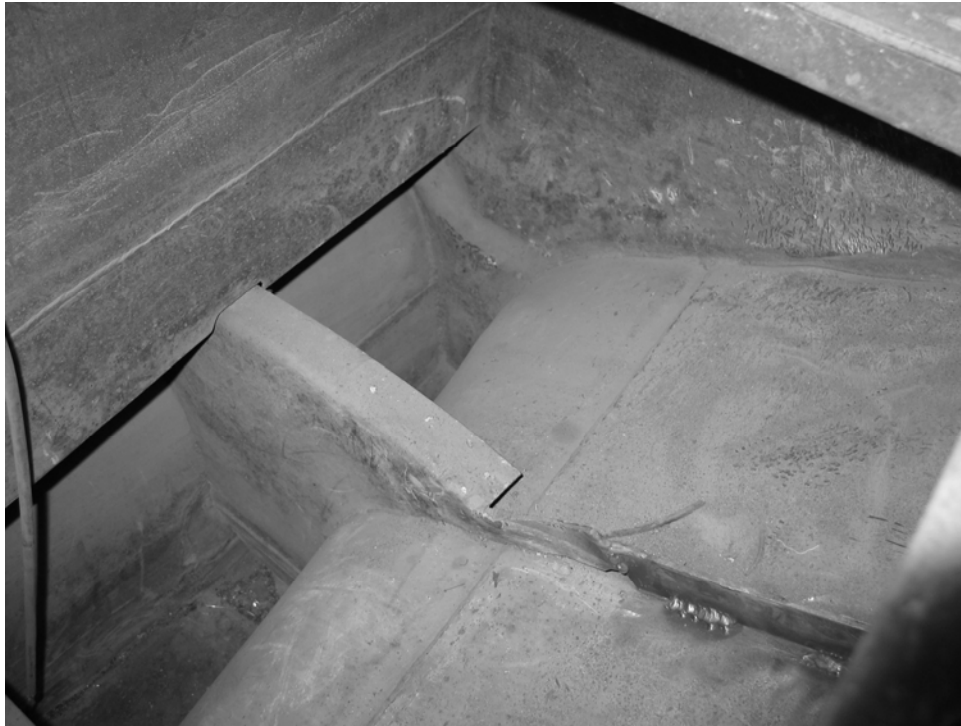
FIGURE 10: Unpainted forward bilge
