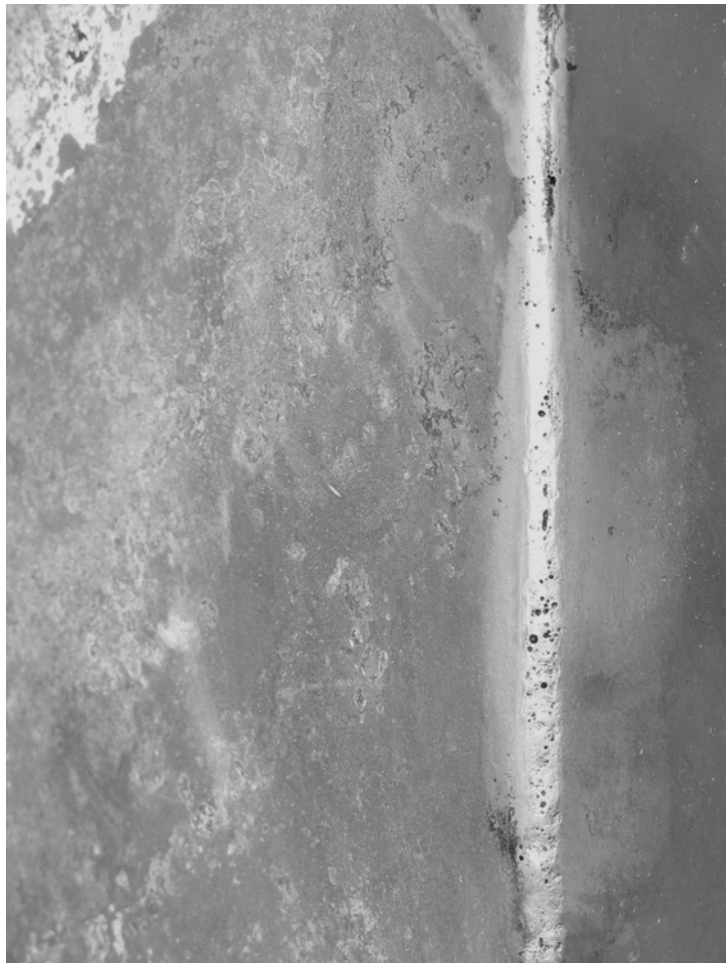
FIGURE 13: Numerous defects in bow weld below the waterline
