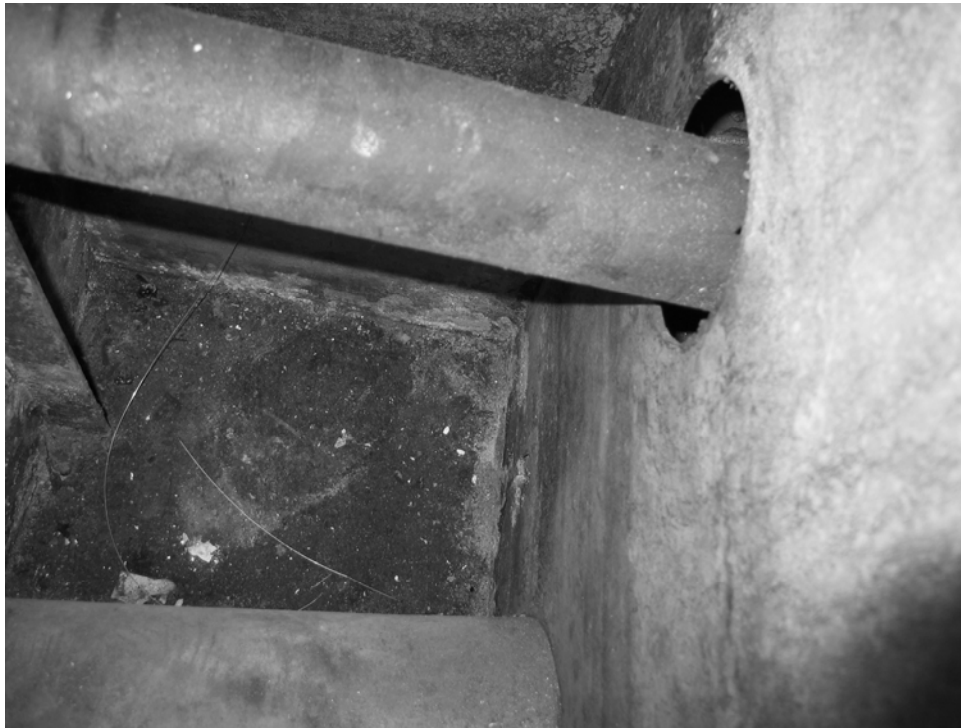
FIGURE 11: Unpainted aft bilge, with shaft passing through, where waste holding tank ruptured
