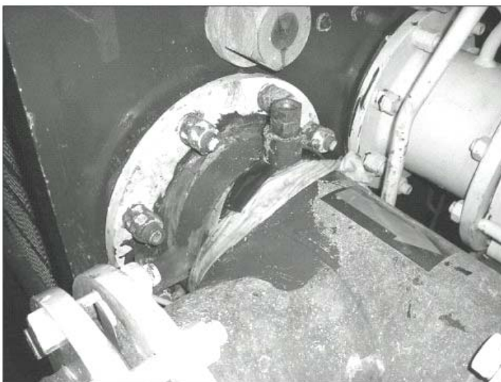
Figure 6: Erosion and galvanic damage behind the welding end at the UNS C70600 outlet pipe of a titanium heat exchanger operated at 4.2 m/s. The pipe and the heat exchanger were not electrically insulated.
