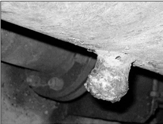
Figure 7: Galvanic corrosion damage of a carbon steel welding end welded directly to UNS C70600-pipe work.
