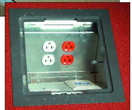
Figure 4. Modular “plug and play” outlets supplied by America Cable Systems, an AFC Company. Top: module with attached cable and connector. Bottom: outlets installed in raised flooring. Electrical specifications call for a maximum of six outlets per branch circuit, a recommended practice intended to reduce the effects of harmonics on sensitive circuits. All branch circuits also have full-sized ground wires. Cable armor, conduit and raceways are grounded but are not used in place of the primary grounding conductor.
