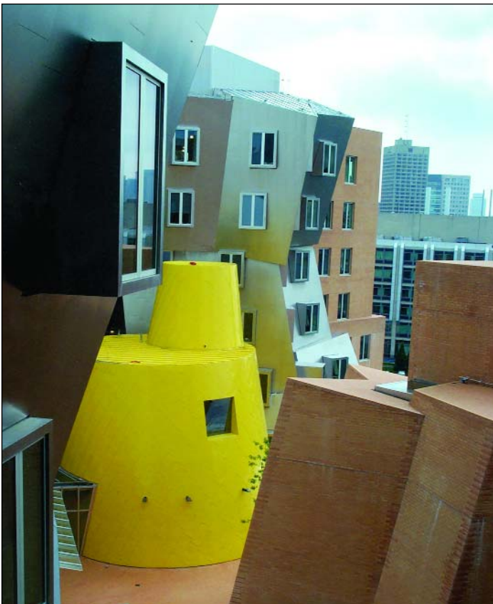
Figure 1. The 720,000-sq ft Ray and Maria Stata Center at MIT, designed by Frank Gehry, is not only one of the most striking architectural works on a U.S. college campus today: it is also a building designed for optimum power quality – an absolute necessity for the sensitive electronic equipment the facility contains.
