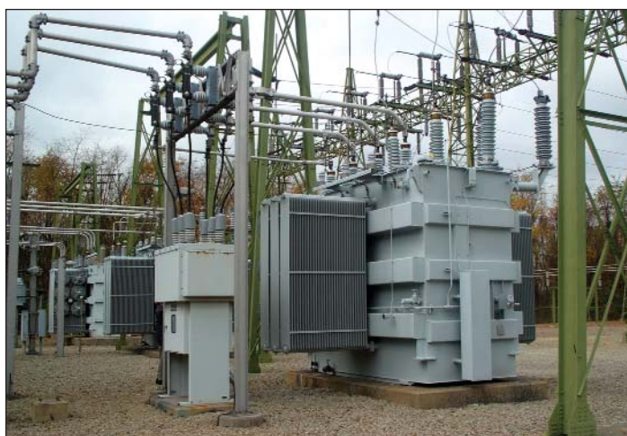
Figure 1. Much of Allegheny Power's distribution system is rural, with radial distribution. In order to ensure long life as well as low lifetime ownership costs, Allegheny Power insists that its power transformers be 100% wound in copper. Reliability is a key factor in transformers of this type.
